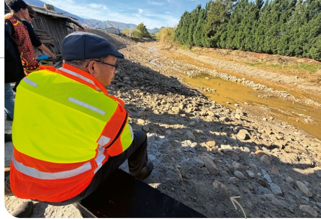
Minister Ivan Meyer assesses flood damage during a visit to affected communities. The floods highlighted the importance of coordinated planning, resilient infrastructure and strong partnerships in supporting recovery.
