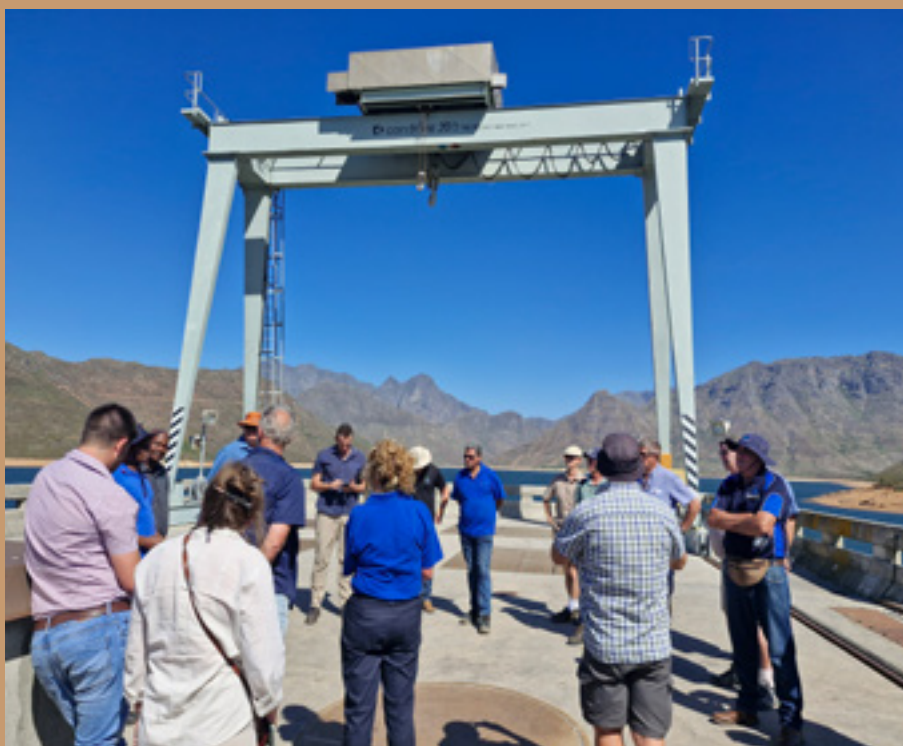
The unique gantry that allows for regular ecological water releases out of the Berg River Dam into the river.
