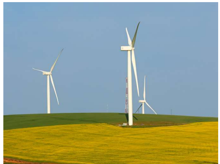
Wind turbines convert the kinetic energy of wind into electrical energy. Photo © Eco Pic
