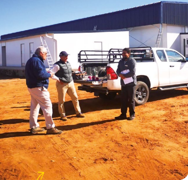
A Veterinary Public Health Official discusses construction of an abattoir at a visit to ensure construction is being done according to the approved drawings.
