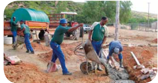
Building a loading area for the ostriches.
